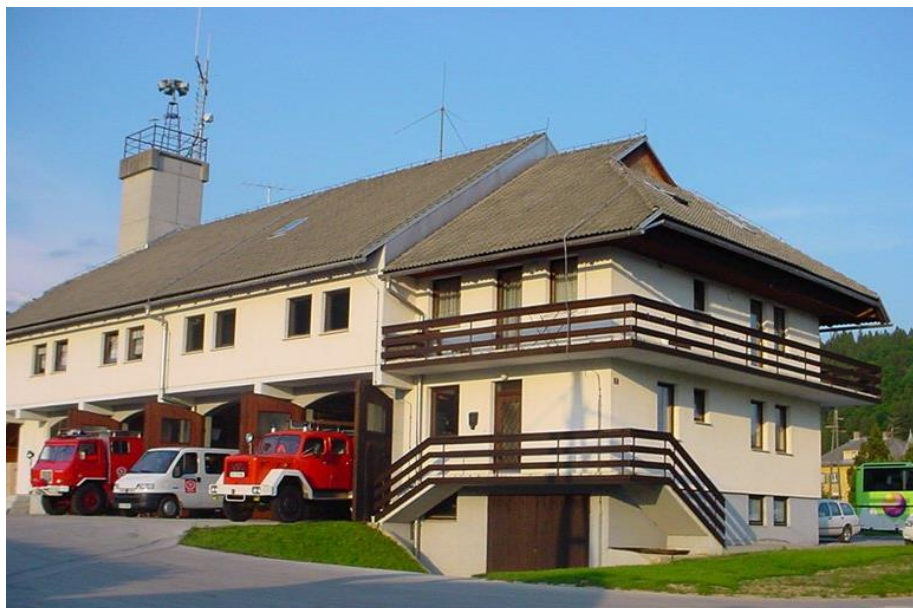
Gasilski dom Begunje Vir: gasilci.org
