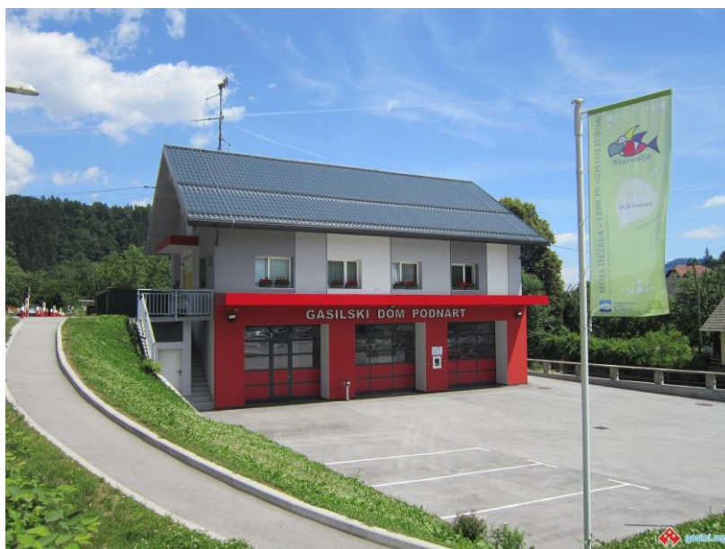
Gasilski dom Podnart Vir: gasilci.org
